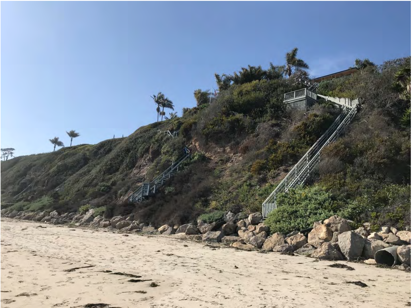
Revetment Adjacent to Pre-Historic Landslide – Sea Ledge Lane (near CoSMoS Transect 4031)
