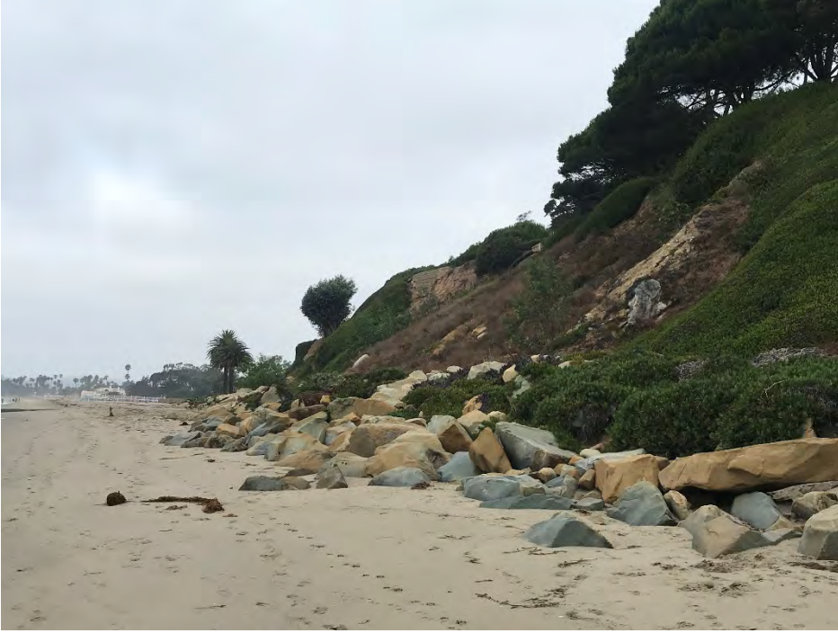
Seacliff Showing Revetment at Toe – View to West (near CoSMoS Transect 3932)
