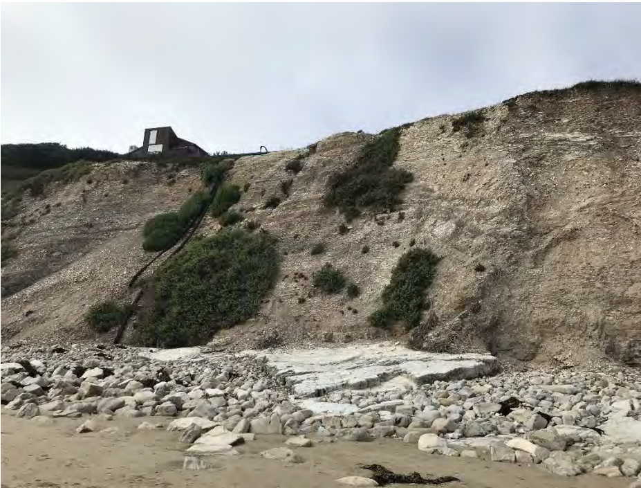
- Ruptured Shale at Toe of 1978 El Camino de la Luz Landslide (near CoSMoS Transect 4001)
