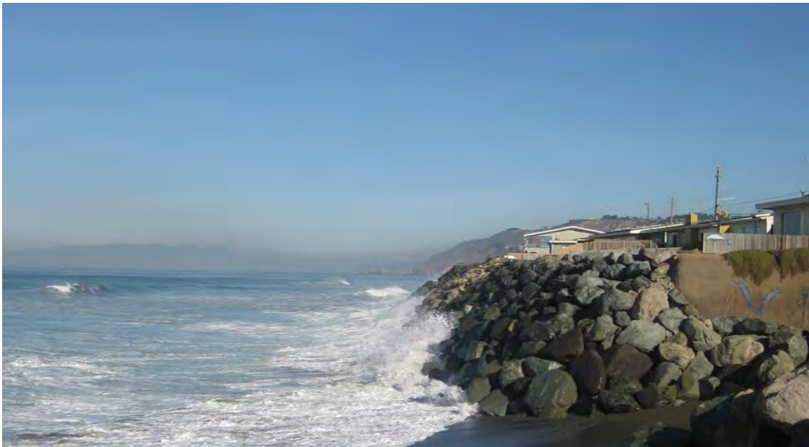
Figure 5-7 Photo of waves against a revetment in Pacifica, CA
