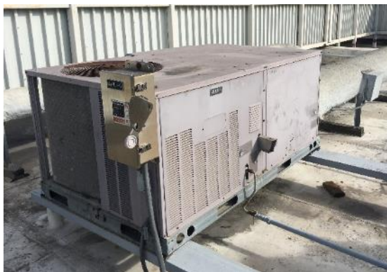
Figure 18: Existing El Estero WWTP Package Unit Proposed to be Replaced
