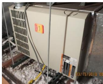
Figure 21: Existing Fire Station 3 Furnace Proposed to be Replaced
