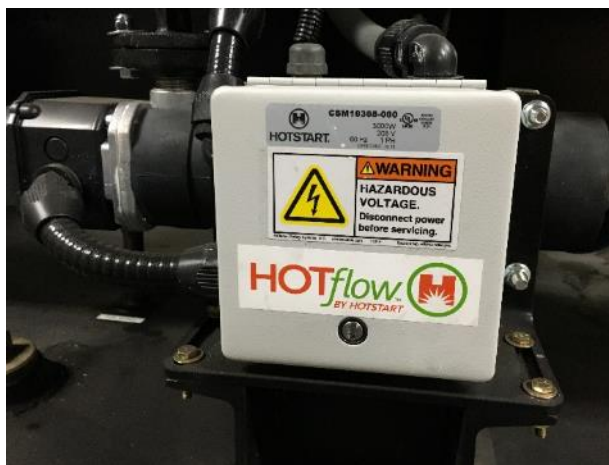
Figure 16: Representative Proposed Circulating Block Heater
