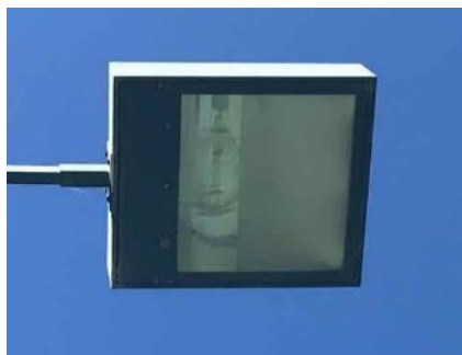
Figure 8: Existing HID Tennis Fixture
