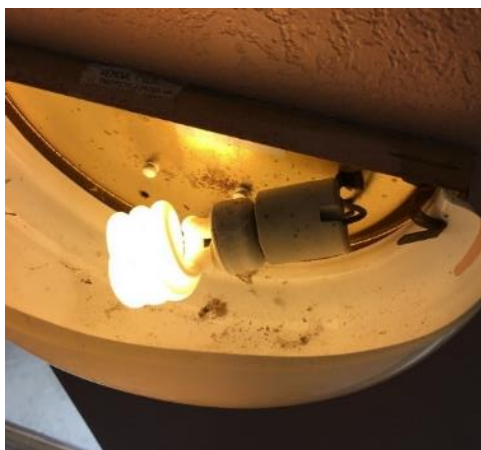
Figure 4: Existing CFL Screw-in Lamp
