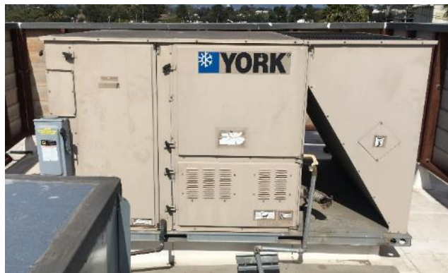
Figure 19: Existing Airport Building 252 (Restaurant) Package Unit Proposed to be Replaced
