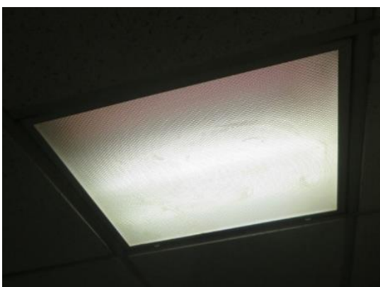
Figure 2: Existing 2x2 Fluorescent T8 Recessed Troffer
