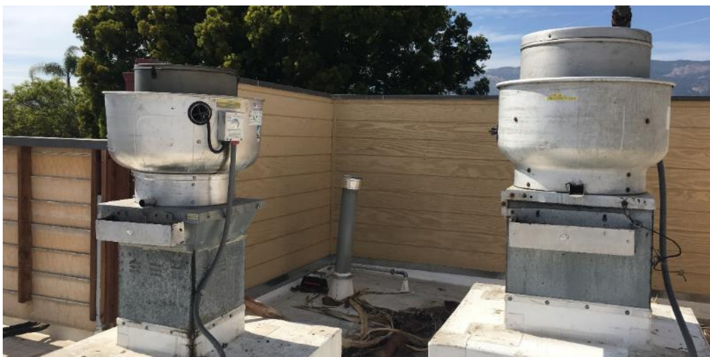
Figure 14: Airport Building 252 (Restaurant) Kitchen Exhaust Fans
