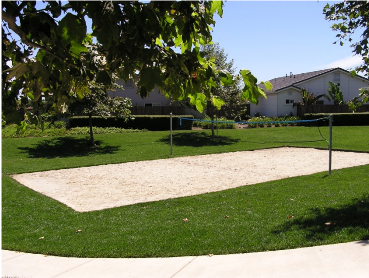
Figure 6-9: Volleyball Court Sand Filter
