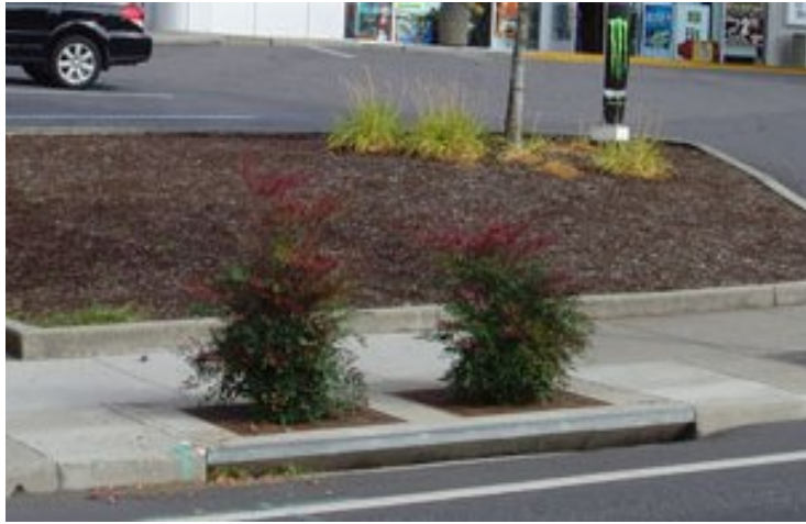
Figure 6-33: Filterra Tree Box Filter
