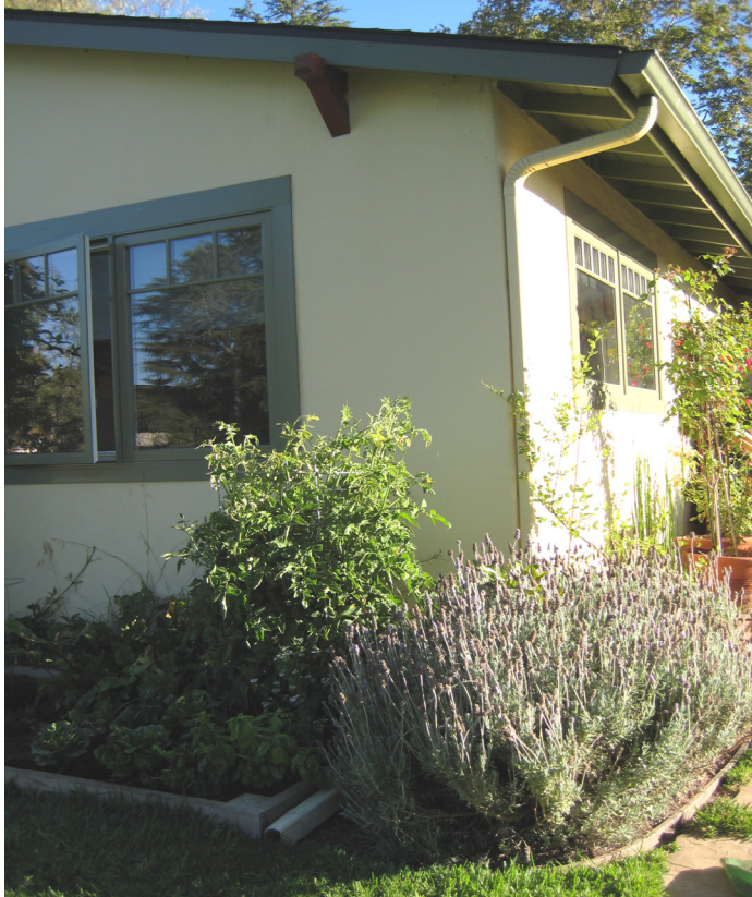
Figure 5-1: Example of disconnected downspout that directs runoff to pervious area
