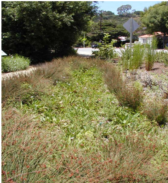
Figure 6-1: Bioretention Area –Arroyo Burro Estuary Restoration Site
