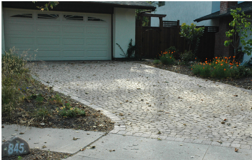
Figure 5-8: Permeable pavers in a driveway in front of a single-family residence in Santa Barbara.
