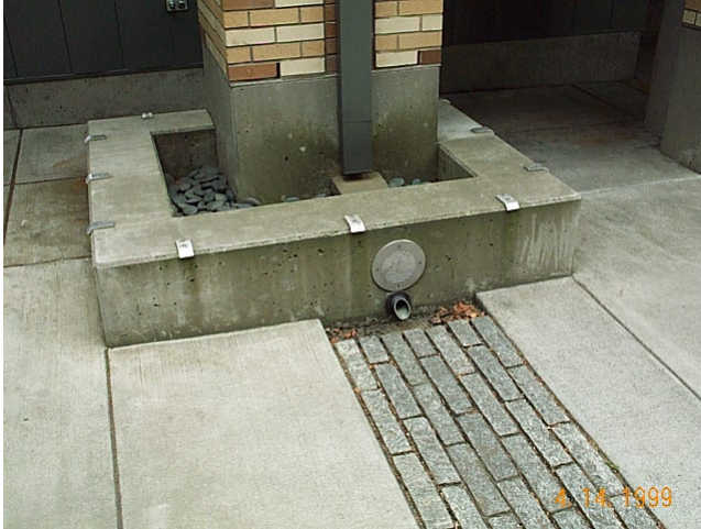
Figure 4-4: Disconnected Downspout Directed to a Pervious Area
