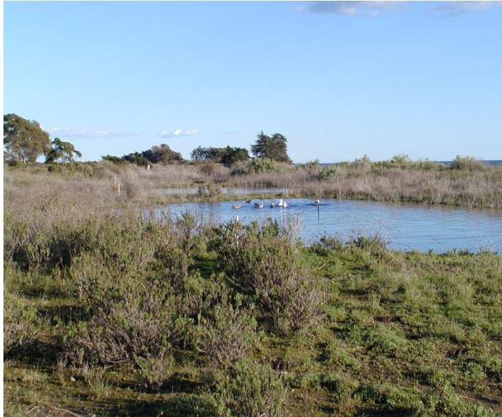
Figure 6-23: Wet Retention Basin with Vegetation Along Perimeter
