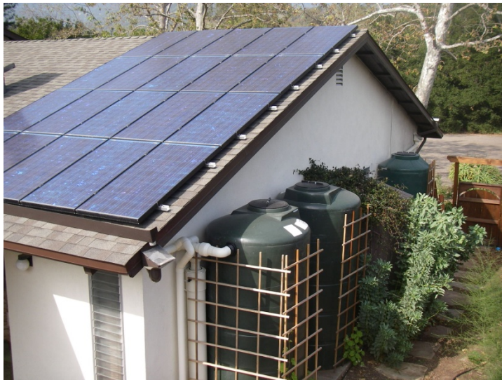
Figure 6-17: Typical Above Ground Cistern
