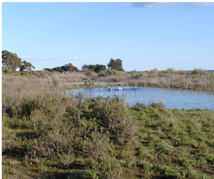
Figure 6-23: Wet Retention Basin with Vegetation Along Perimeter
