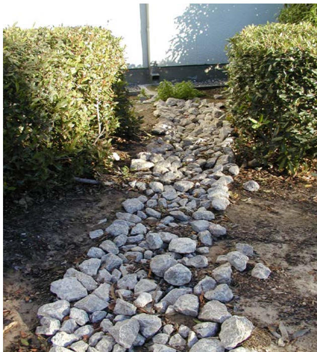
Figure 5-2: Flow Spreading - Directing runoff from a disconnected downspout away from a foundation (University of California, Santa Barbara)
