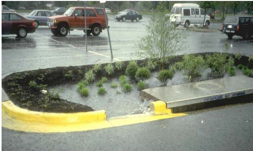
Figure 4-2: Example of minimizing impervious surfaces by implementing bioretention in a parking lot
