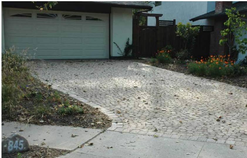
Figure 5-8: Permeable pavers in a driveway in front of a single-family residence in Santa Barbara.
