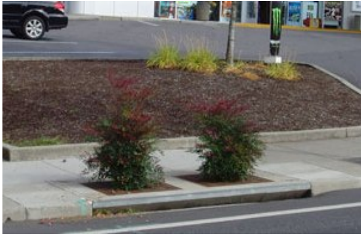
Figure 6-33: Filterra Tree Box Filter
