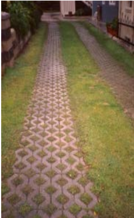
Figure 5-9: Grass paver blocks in a residential driveway
