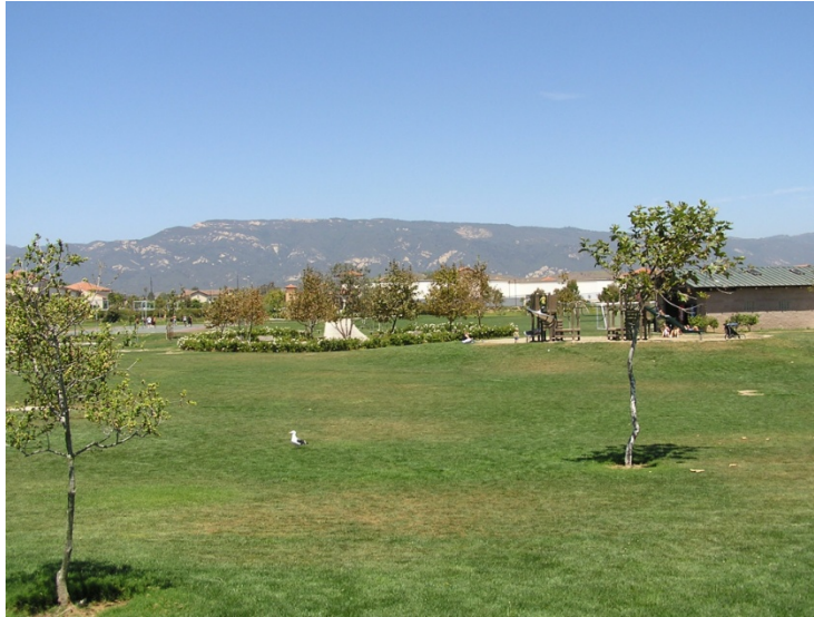
Figure 6-27: Dry ED Basin (dual use; playing field when dry)
