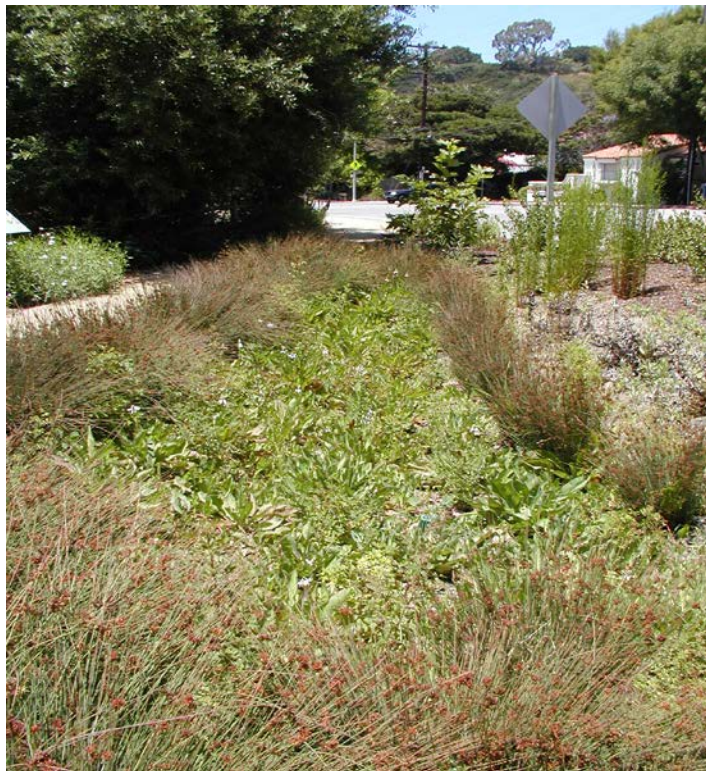
Figure 6-1: Bioretention Area –Arroyo Burro Estuary Restoration Site
