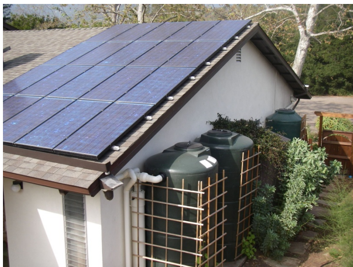
Figure 6-17: Typical Above Ground Cistern
