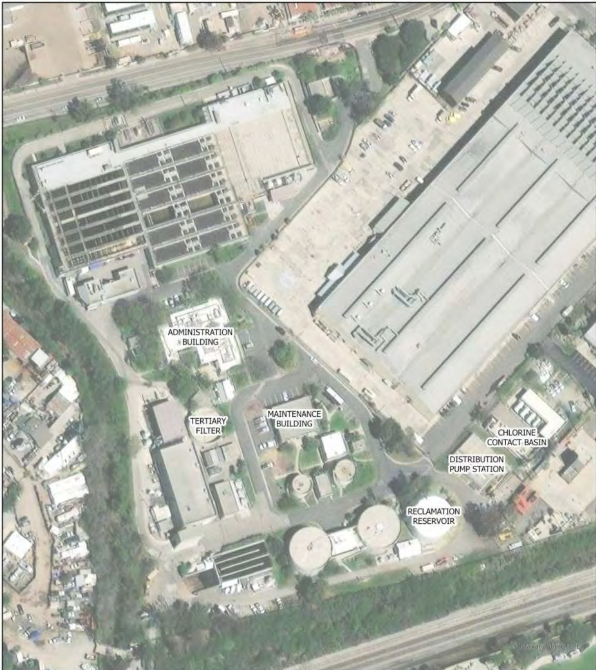
Figure 8-2. Recycled Water Treatment Components [Located at El Estero WRC]
