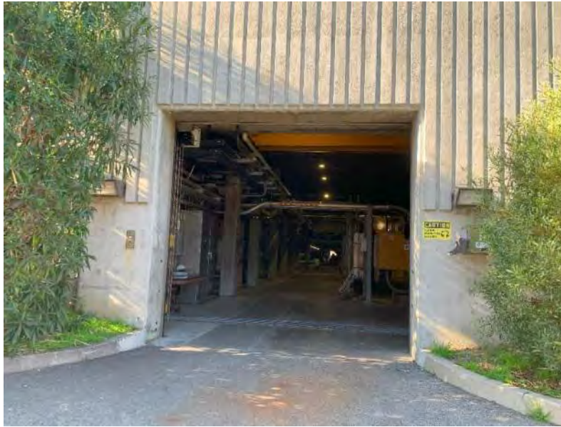
Figure 4-6. Eastern Entrance to Electrical Systems below Aeration Basins (Point 113)
