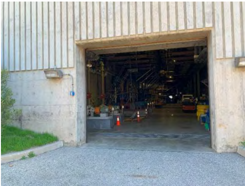
Figure 4-5. Western Entrance to Electrical Systems below Aeration Basins (Point 108)
