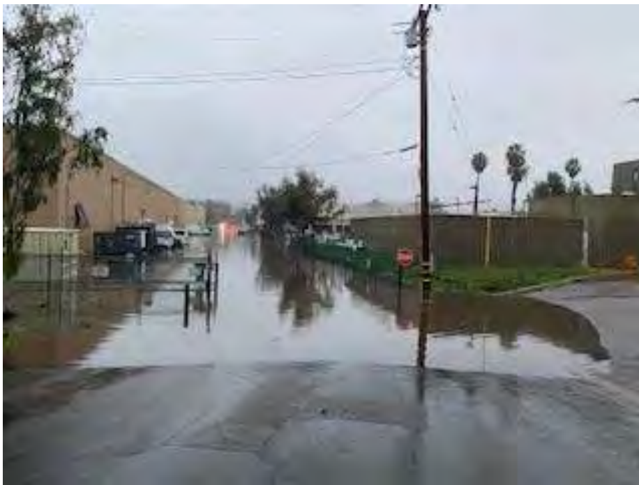
Image Note: Photo taken by City staff at the El Estero WRC back access gate on Quinientos Street during the January 9, 2023, storm (estimated to be a 10-year, 24-hour event). The flood waters are roughly four ft deep at the access gate in this image.
