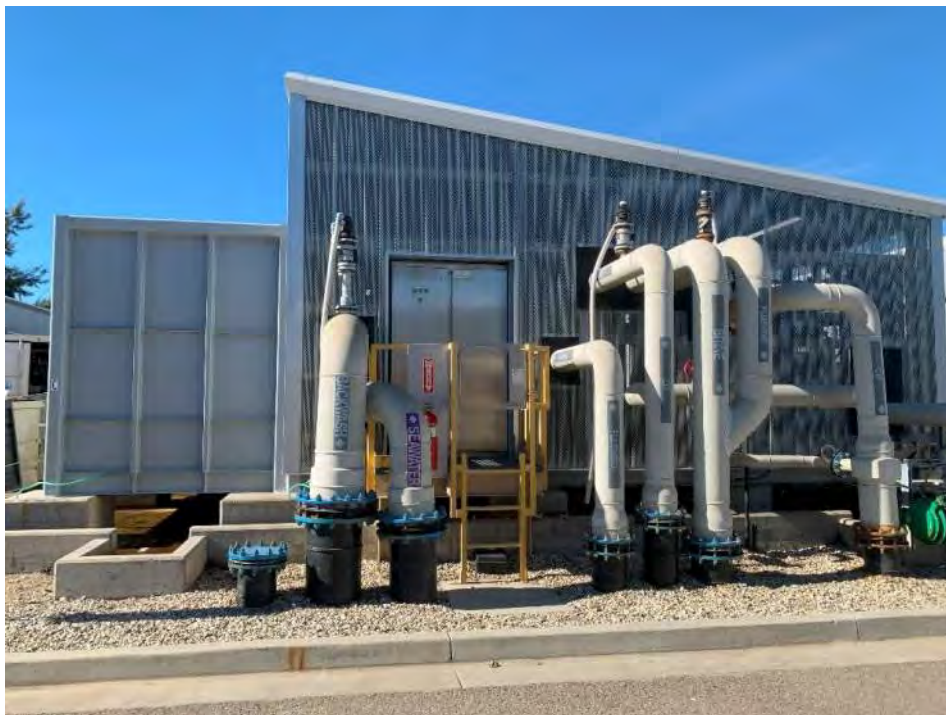
Image Note: Photo of Desalination Plant reverse osmosis modules are 14.2, which is approximately the FEMA base flood elevation plus 1-foot.
