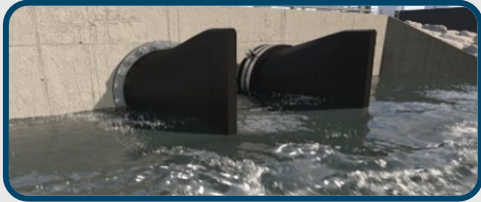
1 Relocate storm drain to improve sand quality
