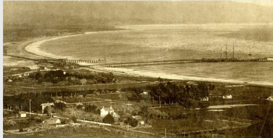
Wharf Spur Construction 1890
