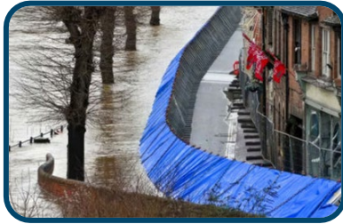
1 Deployable flood proofing
