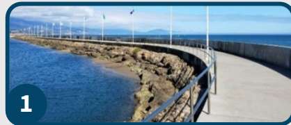
Pedestrian promenade on raised revetment for flood protection & better access
