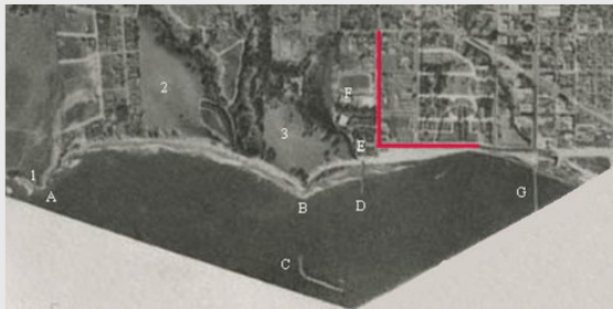
Harbor Under Construction
