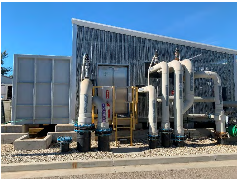
Figure 6-5. Elevated Reverse Osmosis Modules
