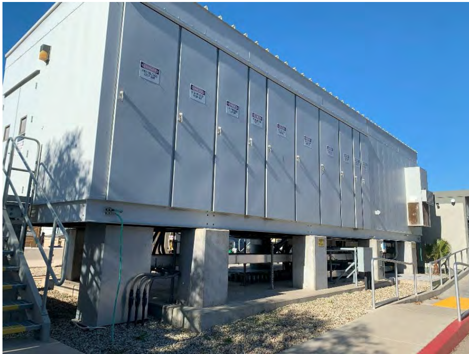
Figure 6-4. Elevated Electrical Equipment at Desalination Plant (Survey Point 118)
