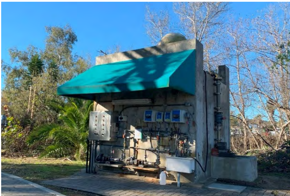
Figure 4-8. Electrical Systems at the Brine Box
